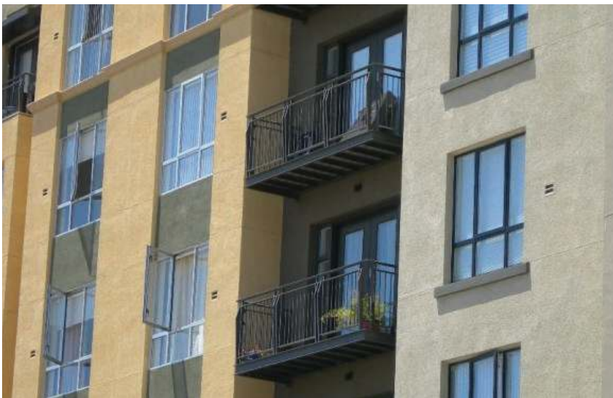
Guideline 5.4.4: These balconies are inset into the building and break up the mass of the building.
