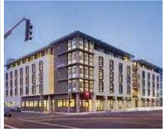
Guideline 7.1.1: Transparency emphasizes the intersection on this building.
