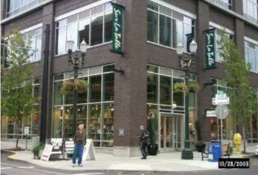
Guideline 4.2.2: Vertical piers and prominent seams provide a vertical break in this facade.
