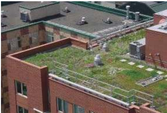
Guideline 6.4: Green roofs filter stormwater
