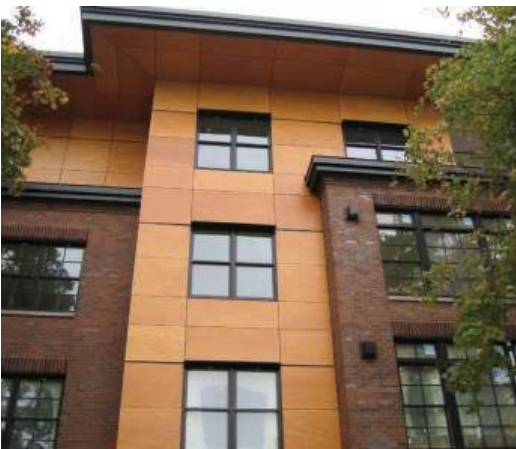
Guideline 6.3: These high density wood composite panels are more durable than traditional wood.
