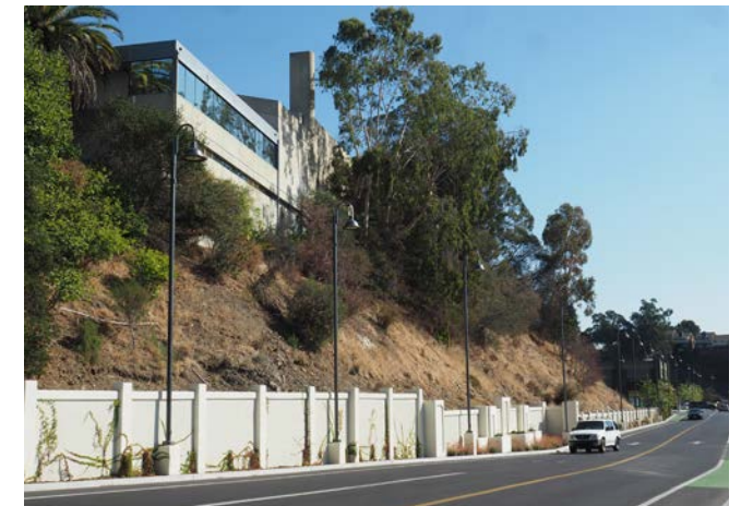
SOUTH SIDE OF SITE/ ACCESS ROAD TO SHOPPING MALL
